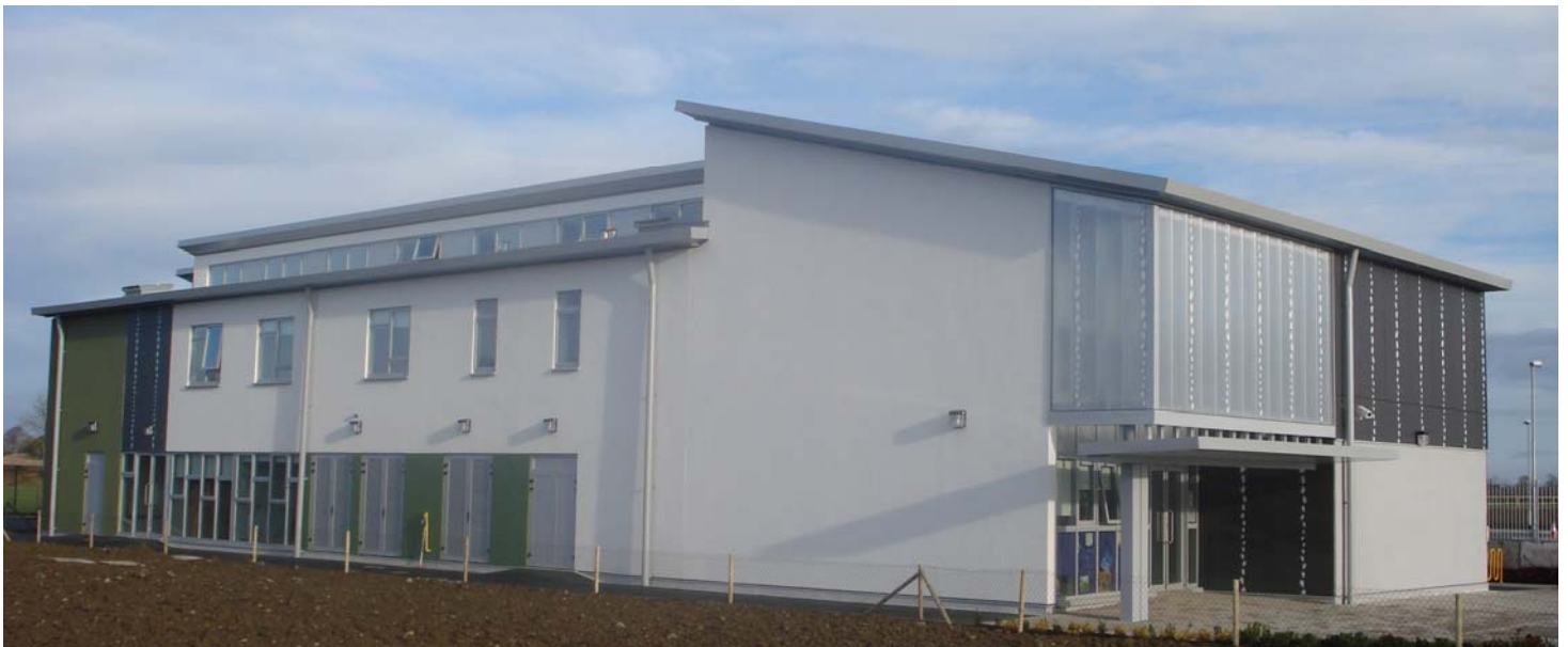
Image 1- View of West Elevation
