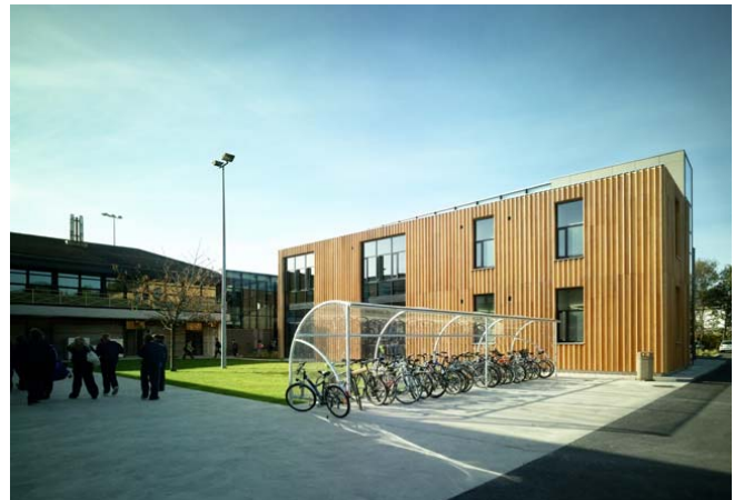
Image 2 - Showing rear larch-clad elevation
