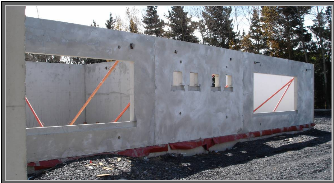
Image 3 - Image indicating precast wall system at ground floor level
