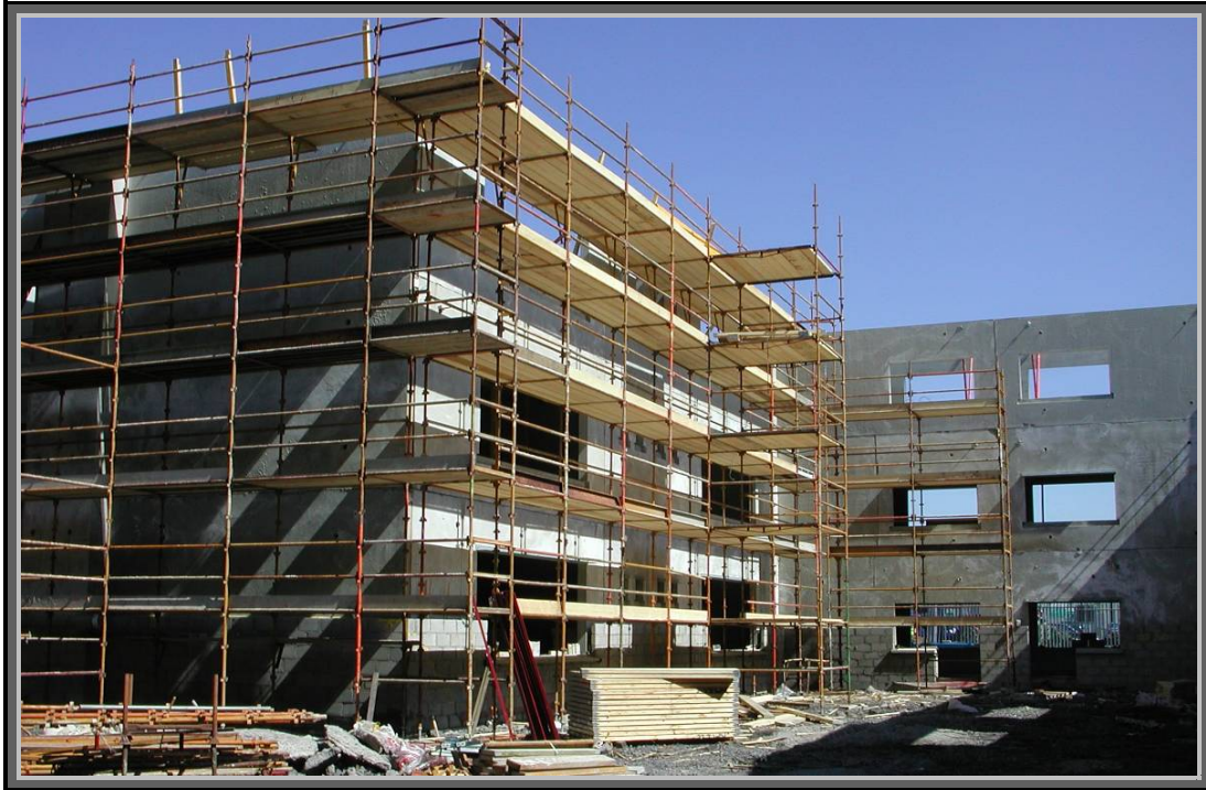
Image 5 - Image indicating precast wall system showing three storeys
