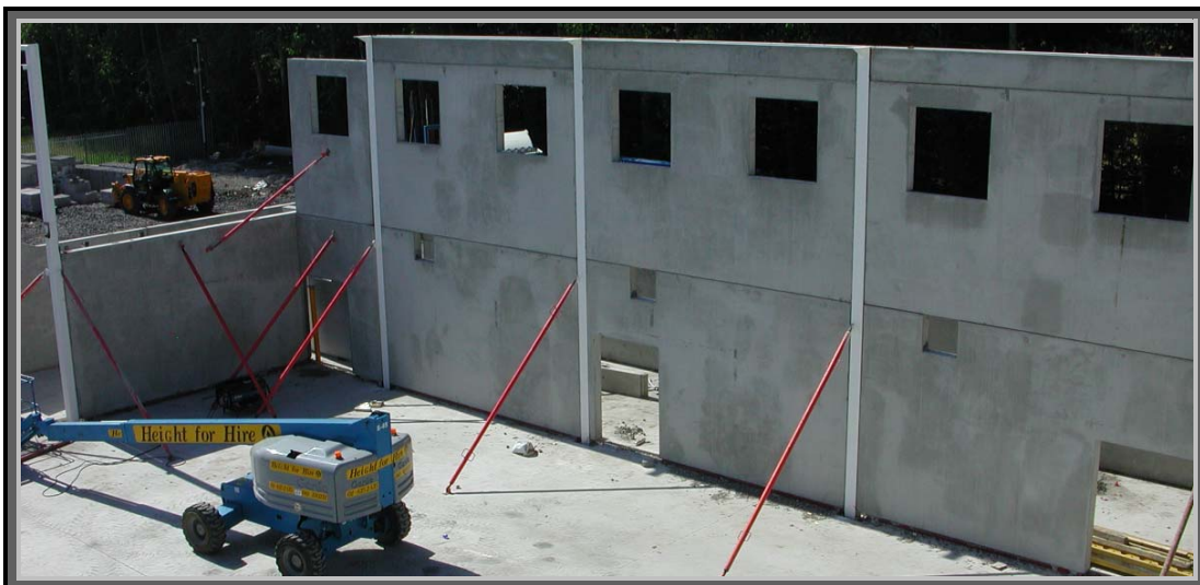
Image 4 - Image indicating precast wall system showing two storeys
